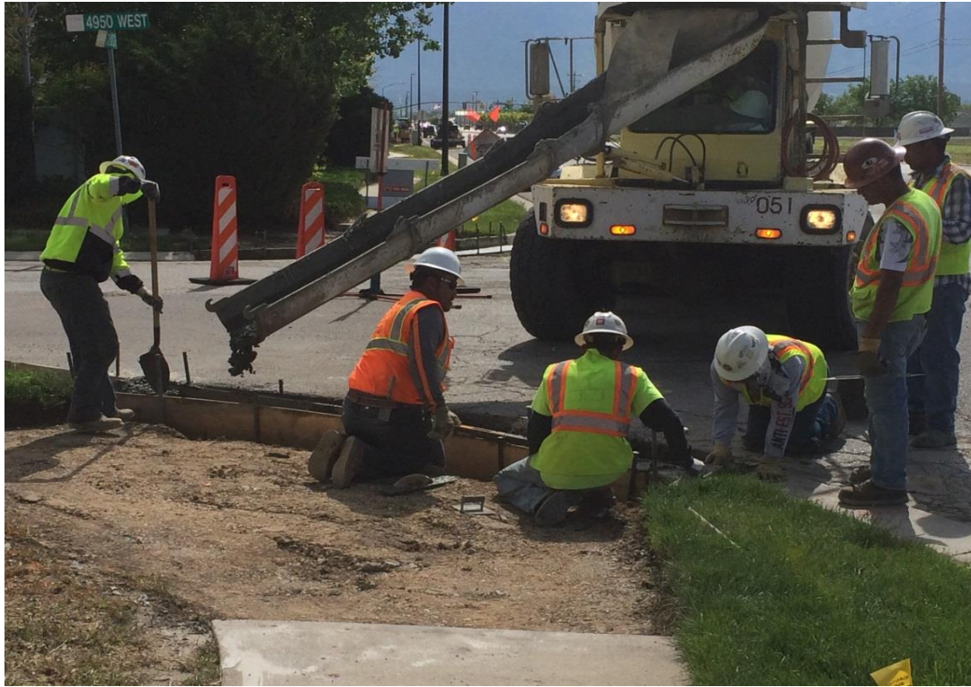
Ramp Construction
